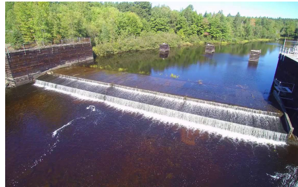
The Narraguagus River ice control dam and timber cribs
